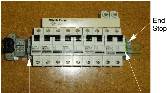
Third End Stop Removed Green/Yellow Block FIG. 10
